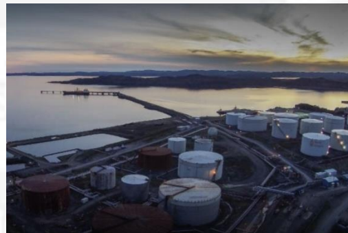
Eight injured in fiery blast at idled Canadian oil refinery, 9/2/2022
