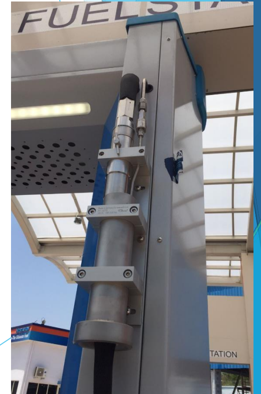
Dispenser-Hose Breakaway Coupling
