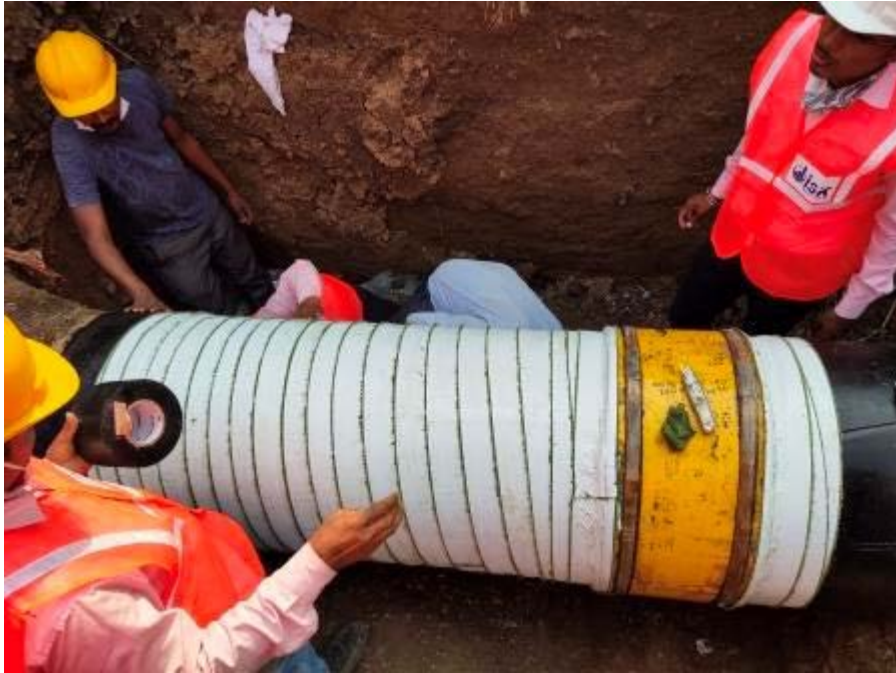
SPECIAL VISCO ELASTIC TAPE & PE OUTER WRAP
