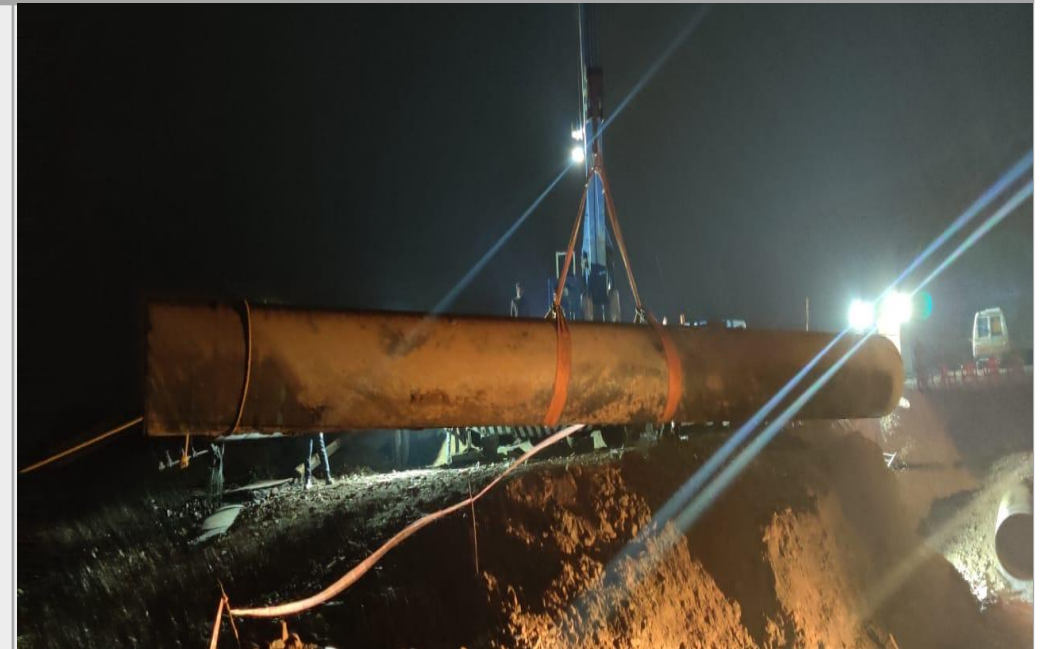
Lowering of Pipe Spool
