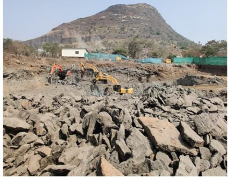
Hard Hilly Strata Cracked
