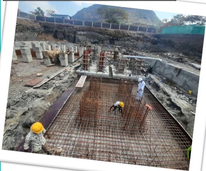
Foundation for 3 rd tank pre-planned
