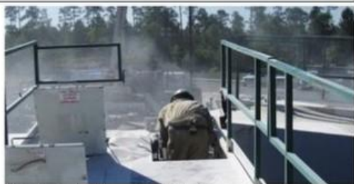
Silica dust cloud by worker delivering sand from sand mover to transfer belt.
