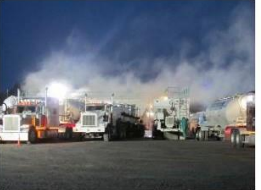
Silica dust clouds from delivery trucks loading into sand movers at a hydraulic fracturing site. Inhalation of this silica is a major hazard associated with oil and gas operations. Image credit: Michael Breitenstein, National Institute for Occupational Safety and Health. 7
