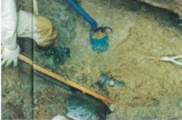
Repairing gas pipe vicinity of damaged water pipe
