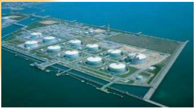
Himeji LNG Terminal (online 1984) 8 LNG tanks, Annual vaporization capacity 6.9 million tons
