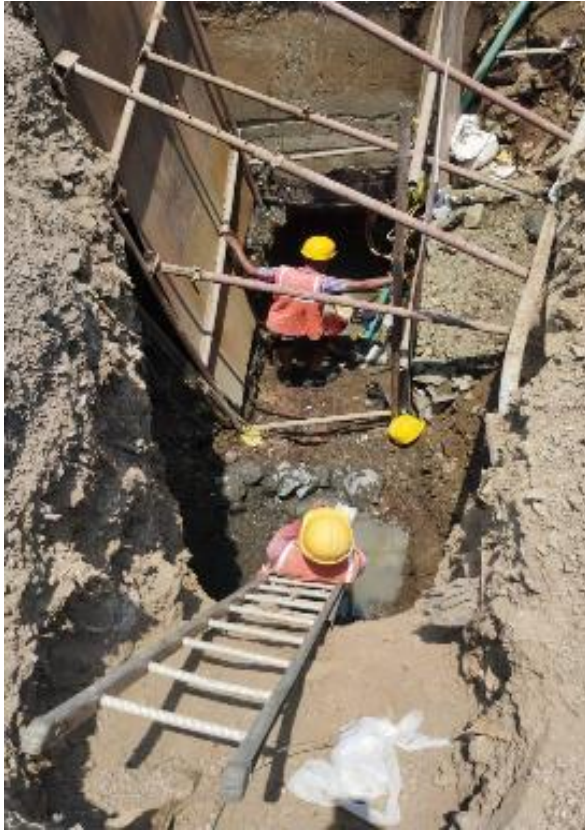
Crossing of culvert at depth > 4 mtrs
