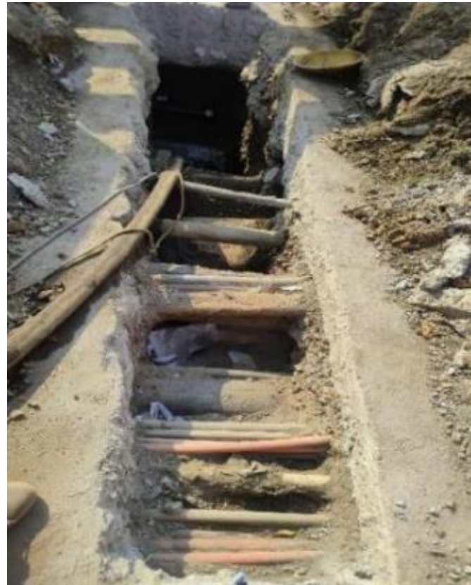
Laying of pipeline amidst cluster of utilities
