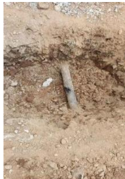
HT/LT cable at shallow depth
