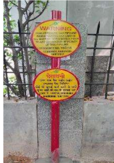
Steel Pole Markers
