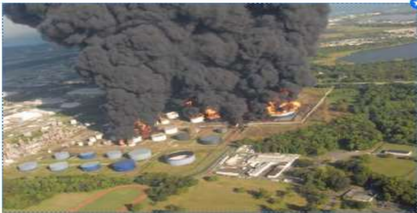
Multiple tanks burning in the fire
