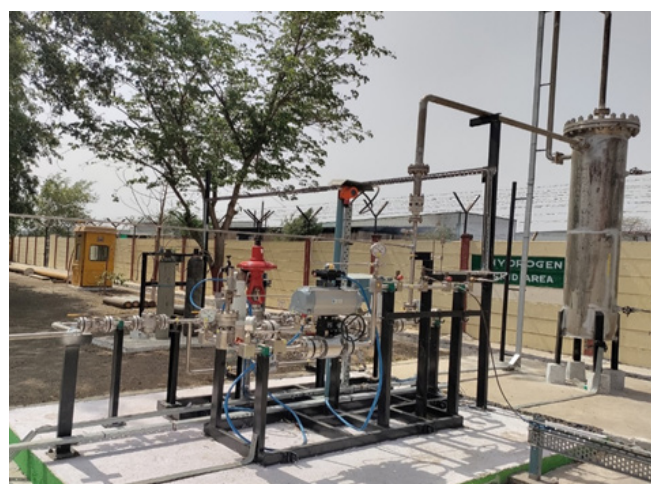
Hydrogen pressure regulation skid at City Gate Station of Indore GA of Aavantika Gas
